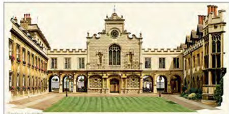
Peterhouse Old Court
